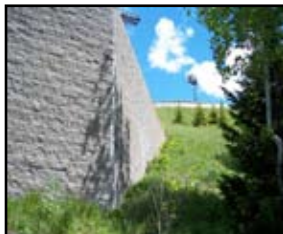
CONTROL TOWER WALL
